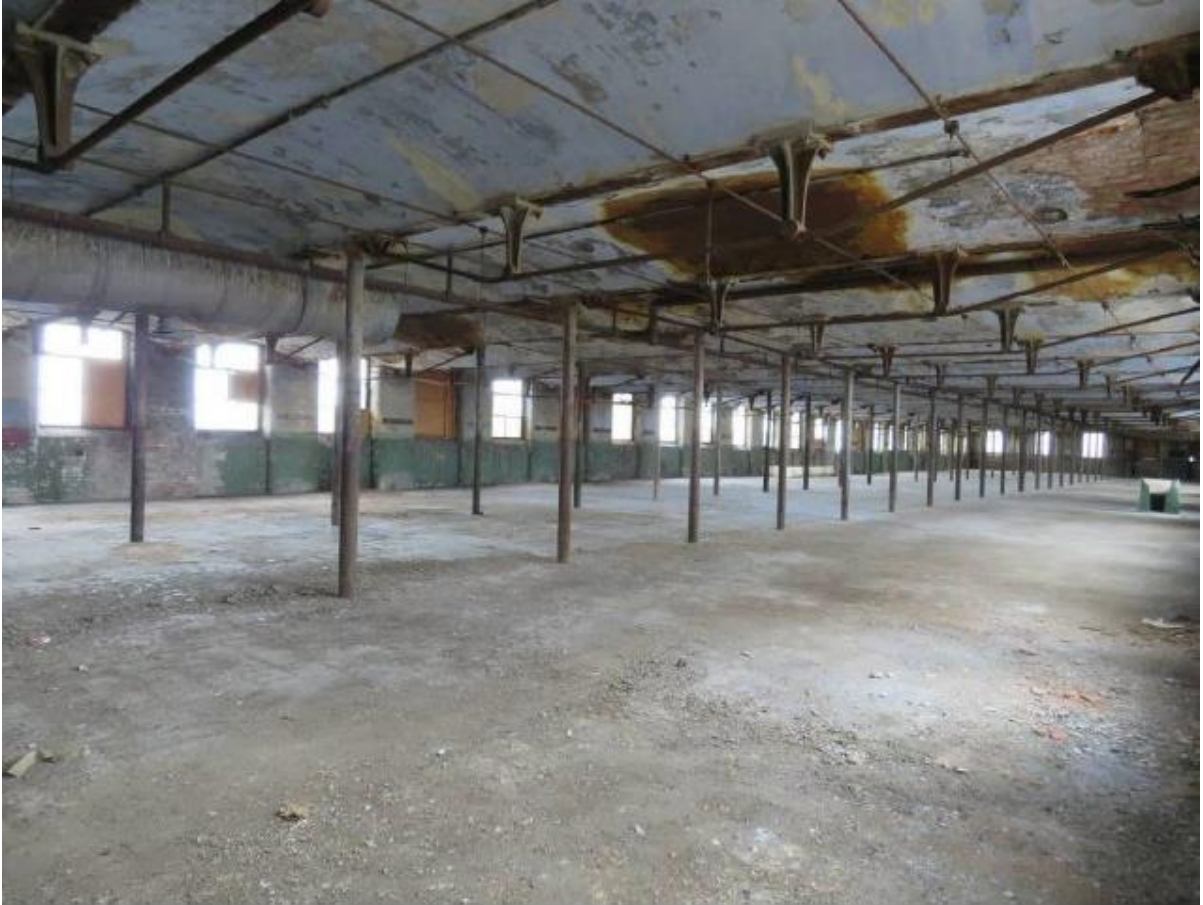
Typical floor layout showing columns and original terracotta quarry tiles
