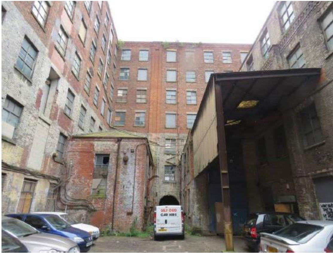
View from within the courtyard including transformer building (left)
